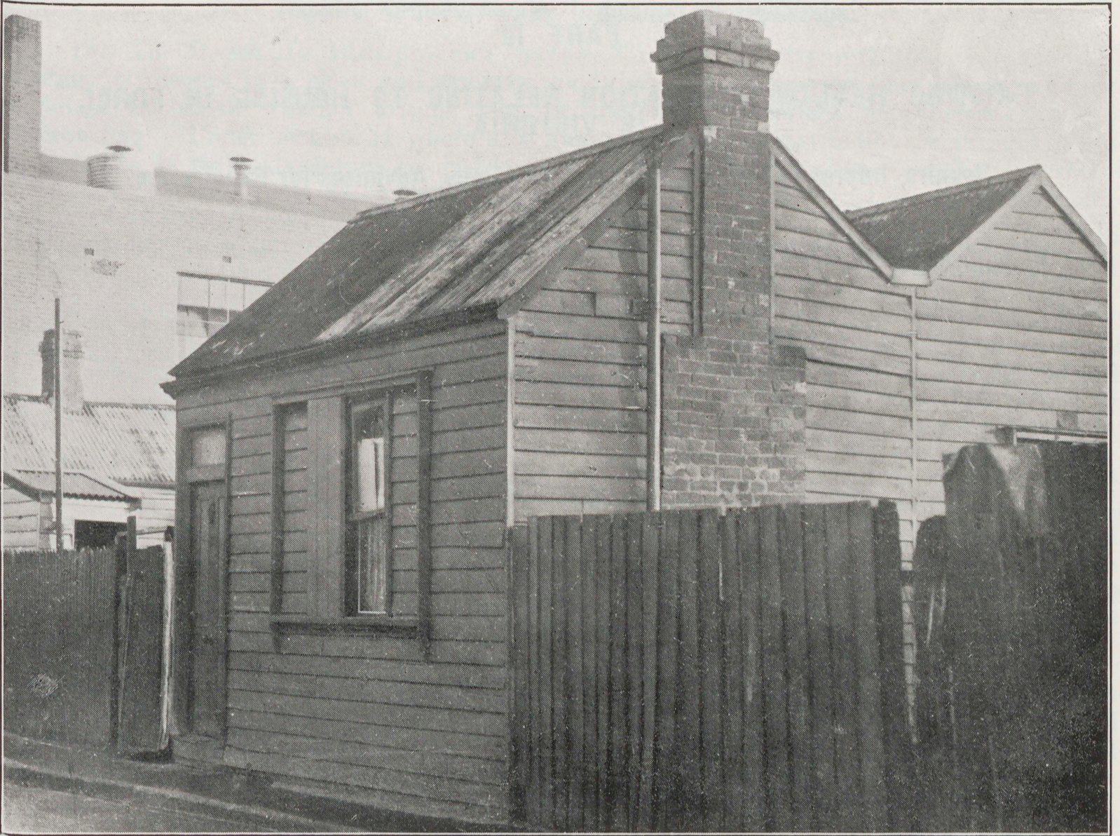
A house in York-street, Collingwood, which is dilapidated inside and out. No repairs have been effected for years and there are no bathing or washing facilities whatever.
