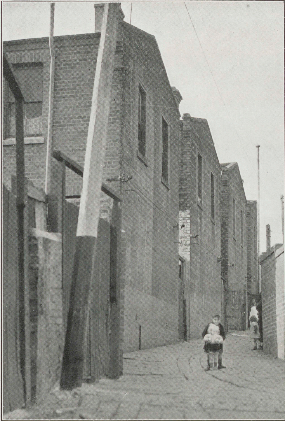
A slum pocket of seven houses where rentals of 12s. 6d. per week are charged. The windows face the narrow alley between each house and receive only 10 minutes sunlight daily. The entrance to each is through the rough wooden gate shown.
