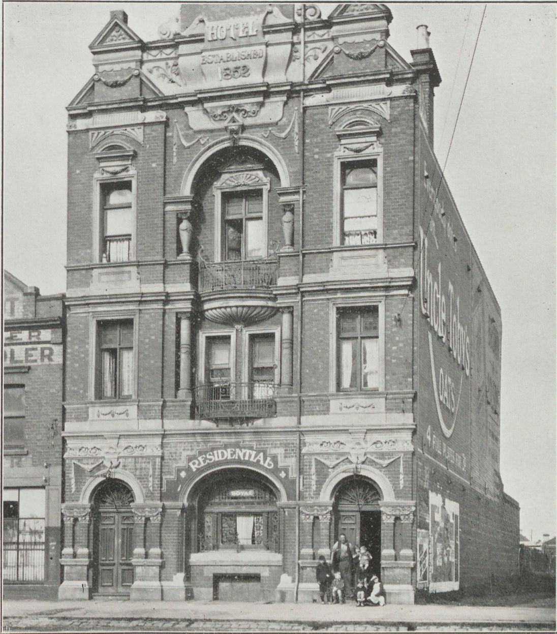
A delicensed hotel at Williamstown. Several families live here in most squalid conditions, with no cooking facilities except open fireplaces, and most inadequate sanitary conveniences.
