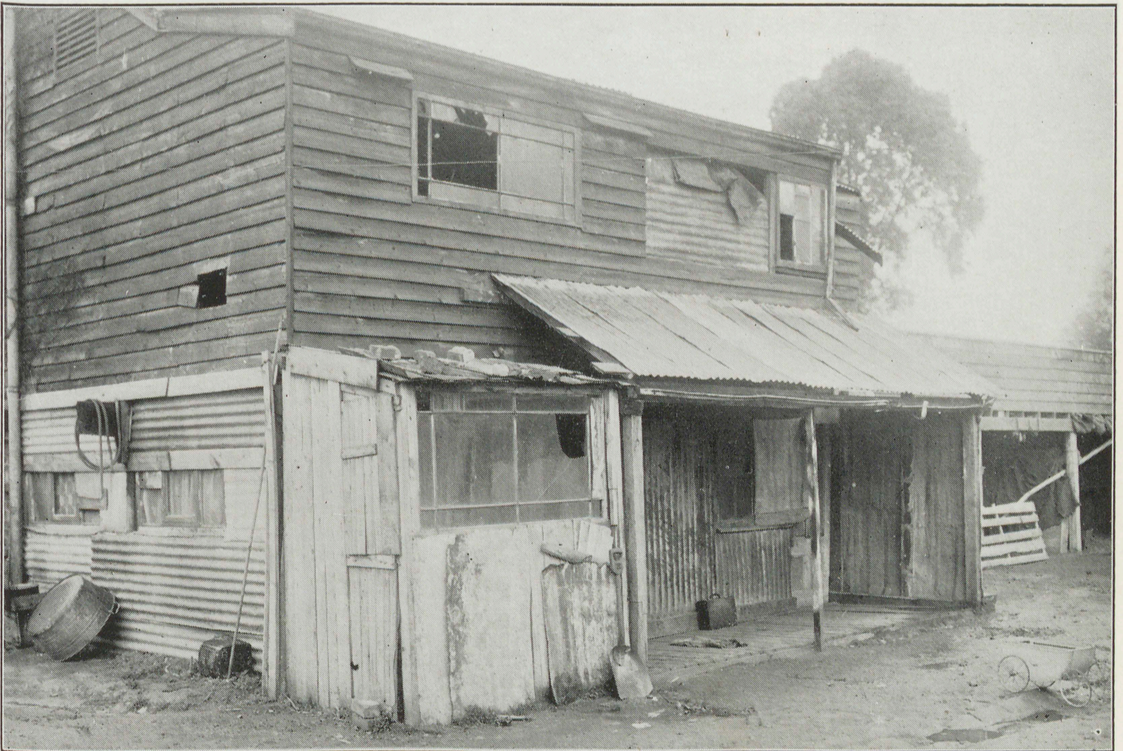
An old factory in Richmond now used as a residence. It adjoins a stable and dumping yard.
