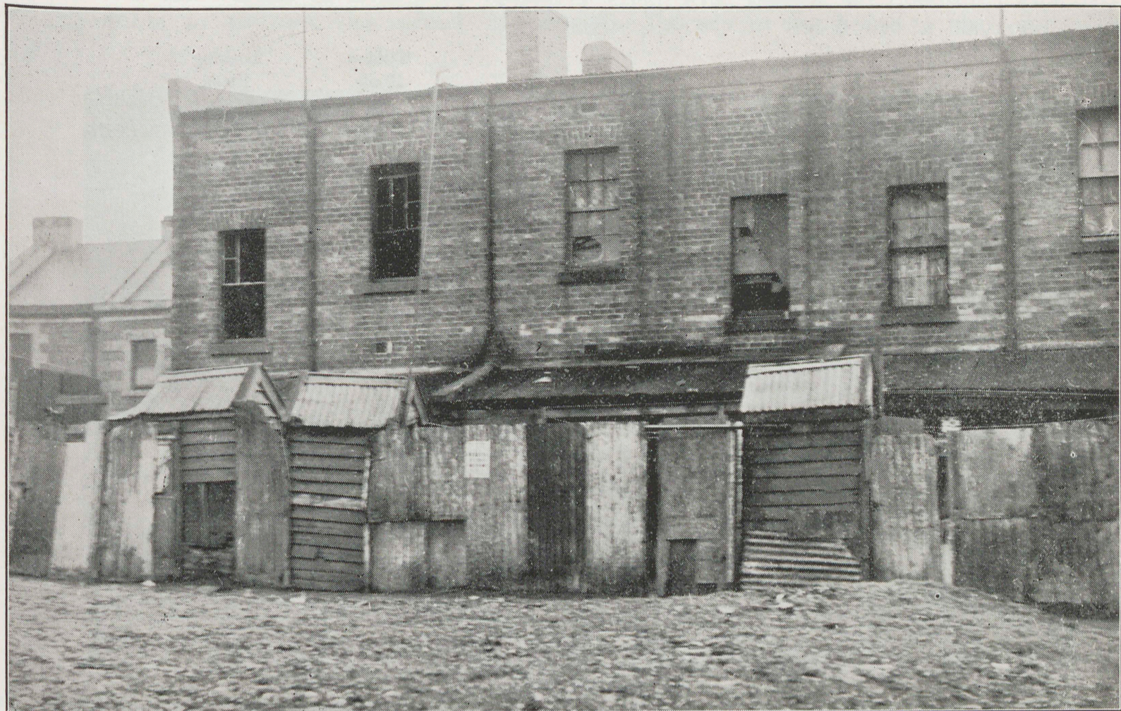
A recent view of premises in Young-street, Fitzroy, showing dilapidated dwellings, fences, and out-buildings.
