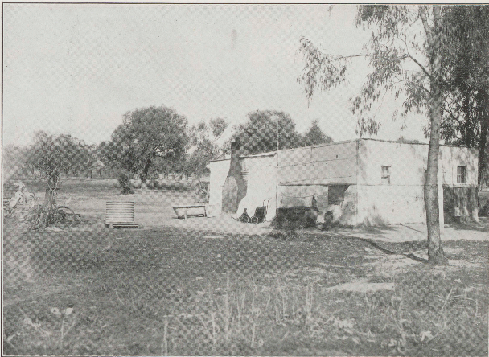
A bag shelter of four rooms in which reside a family of two adults and twelve children. The internal partitions between the rooms are also constructed of bag. This shelter is erected on Crown lands within the boundary of the City of Mildura.
