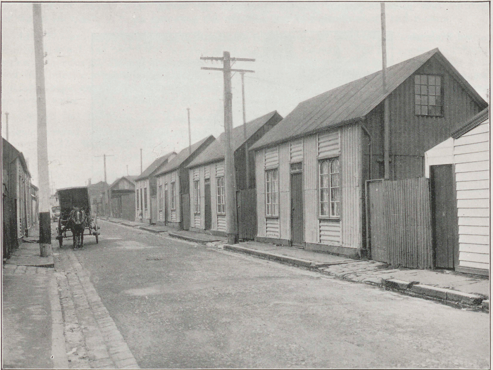
A narrow street of dwellings constructed of iron frames with corrugated iron covering the external walls. These houses were imported in sections approximately 80 years ago. Rentals of these houses range from 8s. to 13s. 6d. per week.
