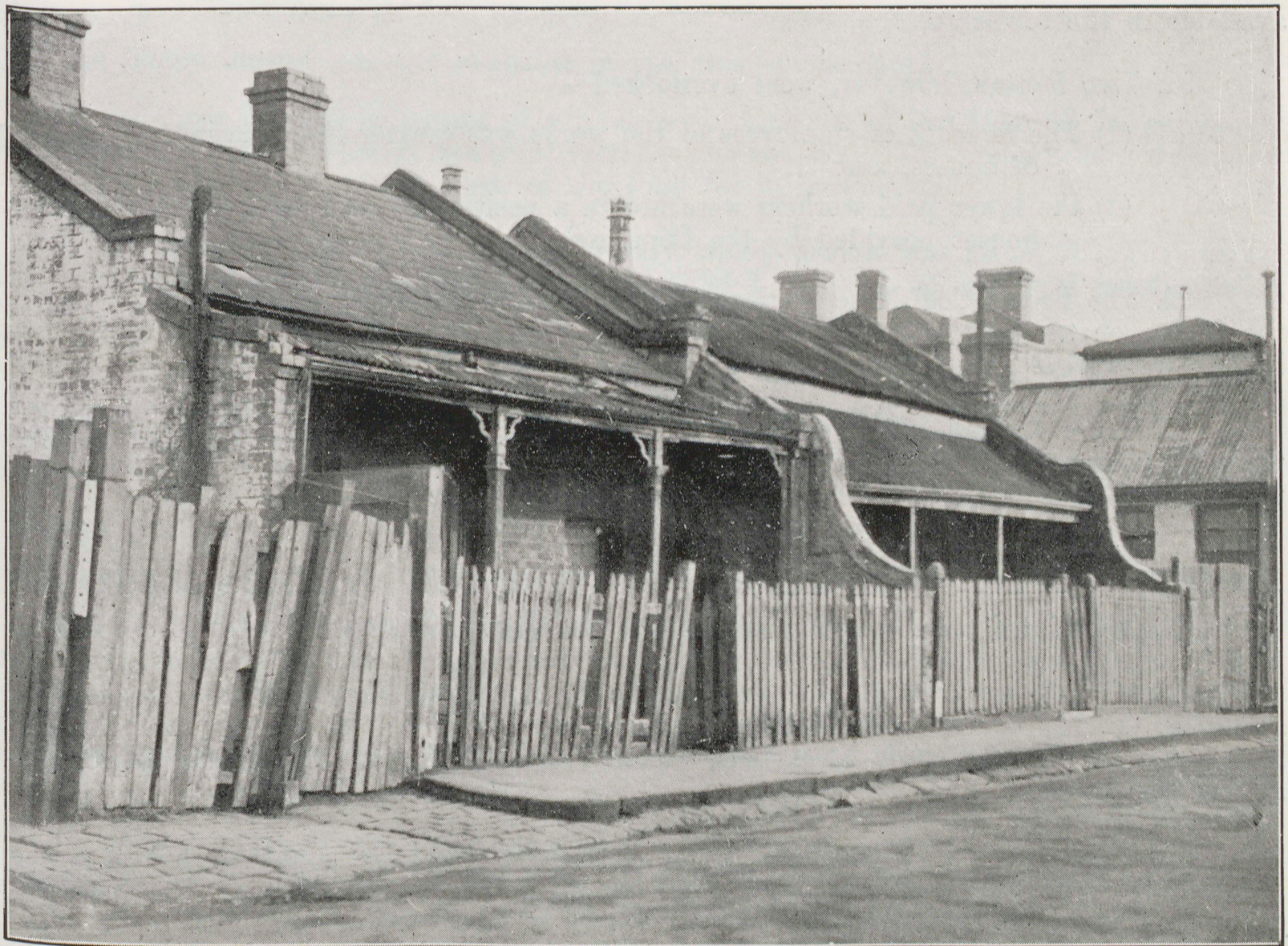
Dilapidated houses in Palmer-street, Fitzroy, for which rentals of 10s. and 13s. per week are charged.
