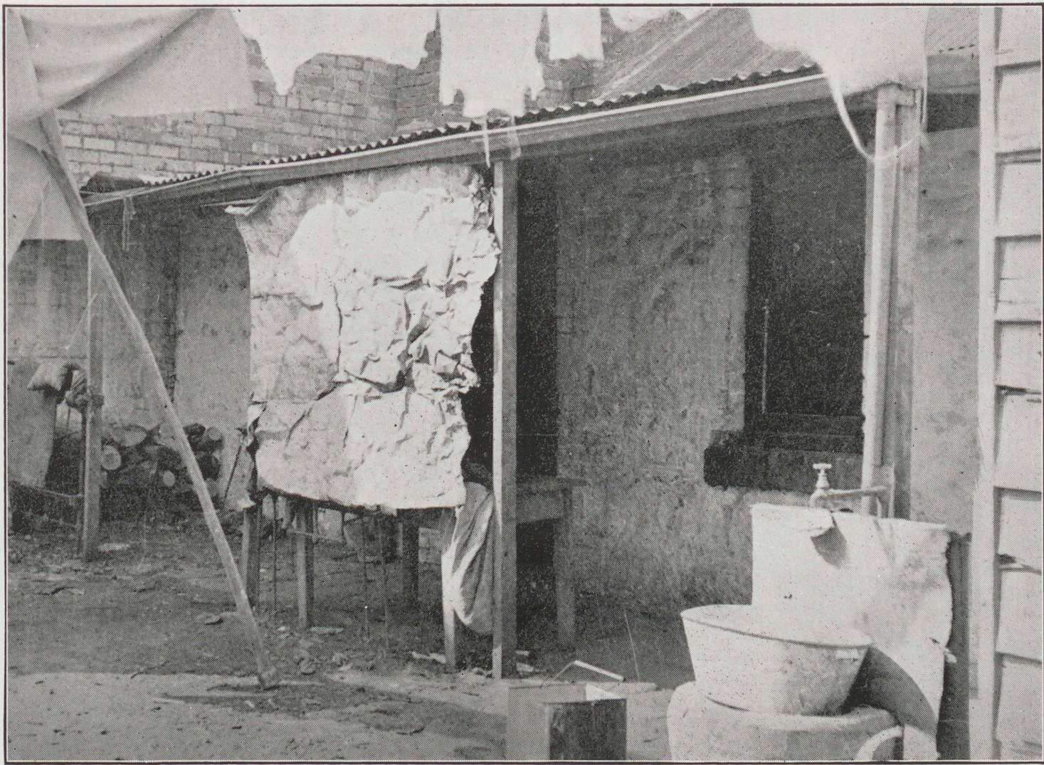
The tub shown is the only bathing facility in this house. The kerosene tin combines the function of bath heater and copper. The tap over the gully trap in the yard is the only source of water supply.
