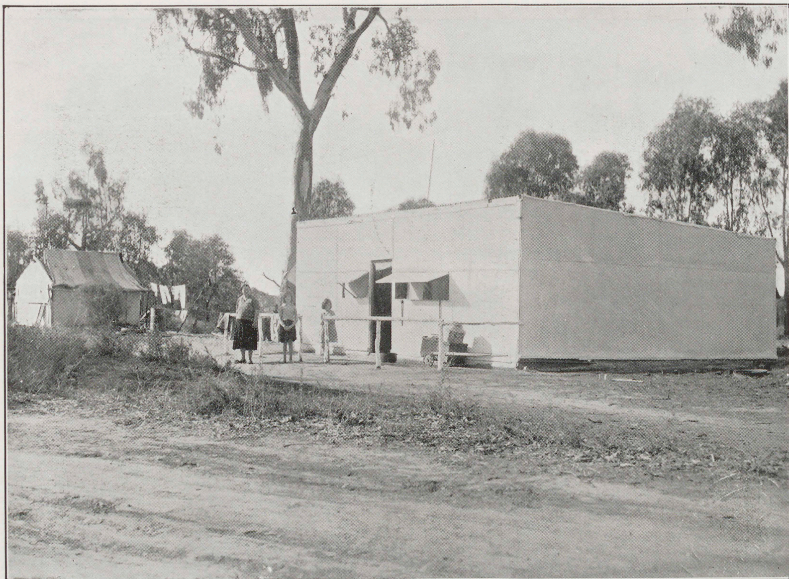
A shelter of timber frame and bag covering. The family in occupation consists of two adults and six children.
