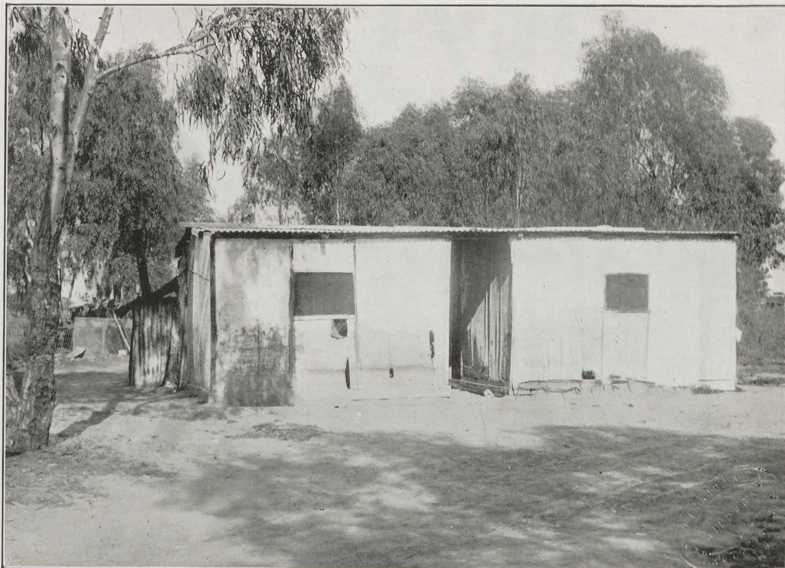
Two adults and nine children occupy this structure with earthen floors.
